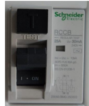
Figure 9: RCCB for the workstation
